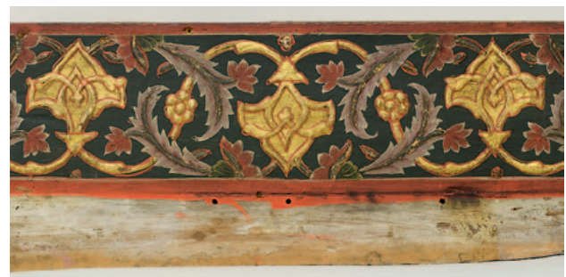
Fig. 5 Detail of 'ataba ceiling panel with gilded and tin-leaved 'ajami against a smalt background. Note the corrosion of the unglazed tin leaf and the discolored smalt; other colors are more representative of the original palette. Image: Mechthild Baumeister © The Metropolitan Museum of Art.
