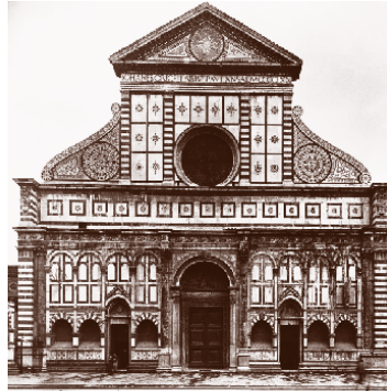
Façade of Santa Maria Novella, designed by Alberti Foto Marburg/Art Resource, N.Y.
